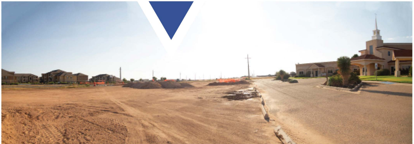
The entrance from 130th St. is now closed and more than half of the front parking lot is being used for construction for Loop 88. Photo taken August 2023.
